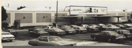
Walthers completes its move to its current home at 5601 W. Florist Avenue on Milwaukee's north side.
